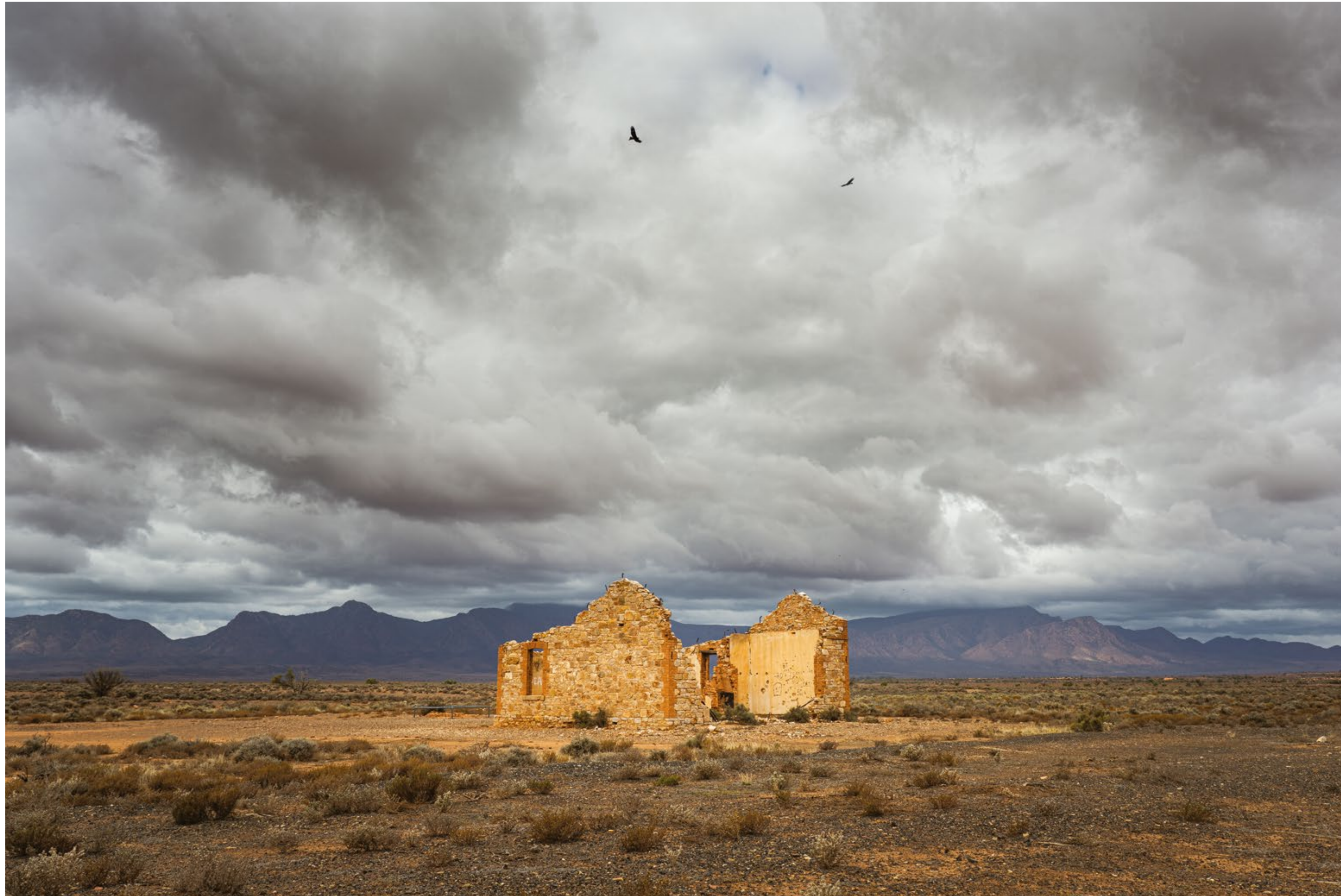
Edeowie Railway Siding \ MP
